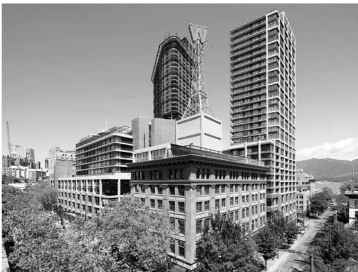
Figure 2. Woodward District, Downtown Eastside, Vancouver. Opened in 2005, the Woodward district occupies a full city block with two towers of market and affordable housing, commercial, institutional (including City government and Simon Fraser University), and recreational space. The development is symbolic of the wager in the City’s “revitalization without displacement” strategy in the DTES, but – ominously for the homeless – also marks the take-off point in rapid condominium development in the neighborhood (photo: John Goldsmith)
